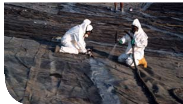
Polyurea being applied to Geotextile fabric for a reservoir liner.
